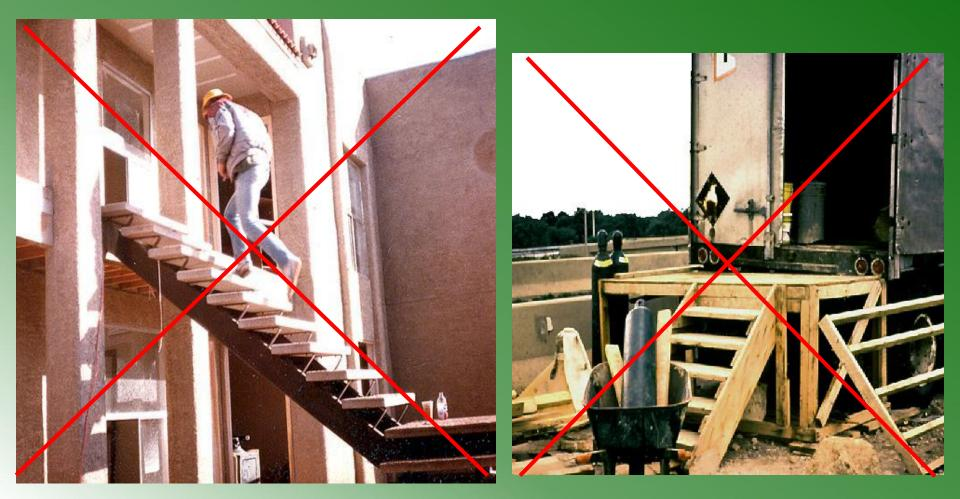
Midrails, screens, mesh, intermediate vertical members, or equivalent provided between the top rail of the stairrail system and the stairway steps.
