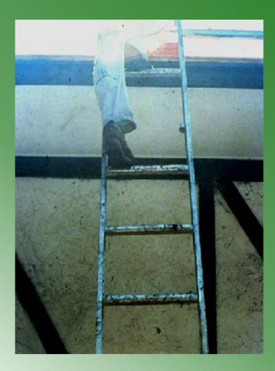
Portable or fixed ladders which are damaged must be taken out of service and tagged "DO NOT USE"
