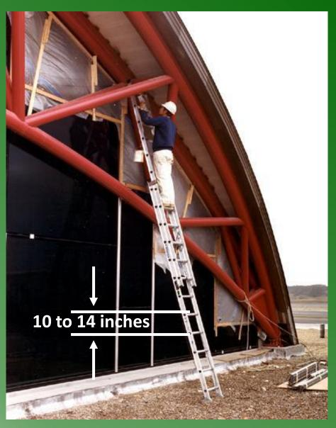
• Rungs and steps of fixed metal ladders & portable metal ladders must be corrugated, knurled, dimpled, coated with skid-resistant material
