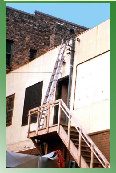
Ladders shall have nonconductive siderails if they are used where the employee or the ladder could contact exposed energized electrical equipment.
