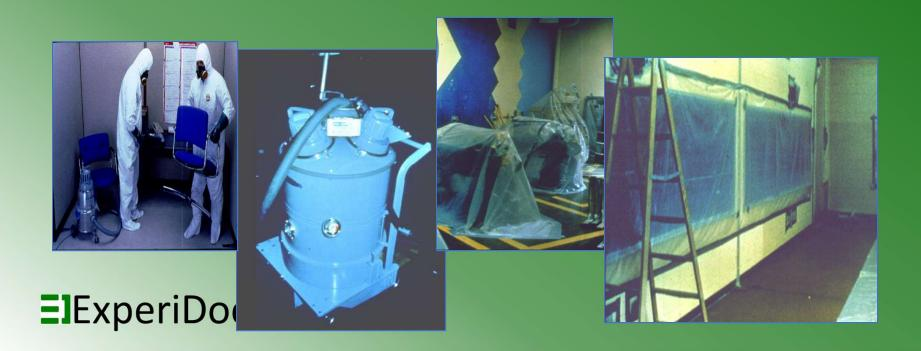
• Construct Plastic Containment – 2 layers 6 mil on the floors & 2 layers 4 mil on the walls.
