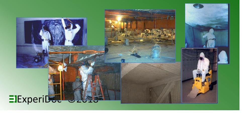
• After Removal, Double Bag debris in (2) 6 mil plastic bags, & Conduct Clean-up.
