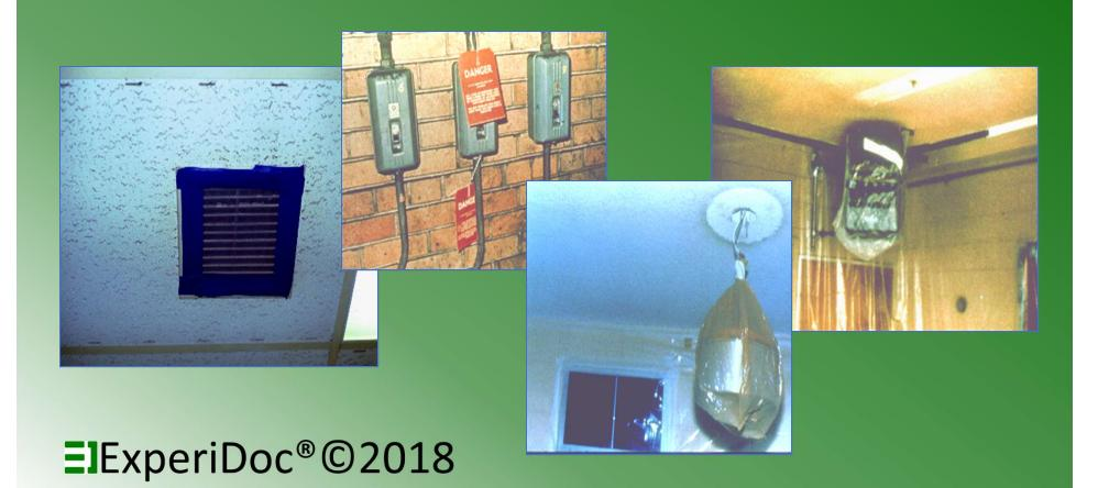
• Preclean all items with wet wiping techniques and HEPA Vacuum. Remove items from the work areacover stationary items with 2 layers 6 mil Plastic.
