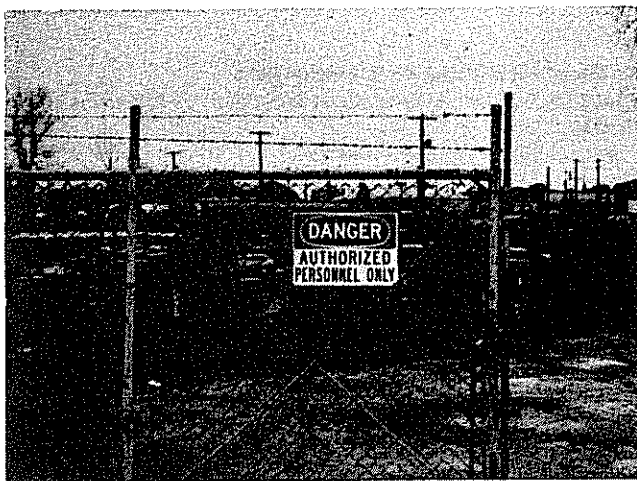
Warning signs and fences help to prevent exposure of unauthorized and unprotected people to site hazards.
